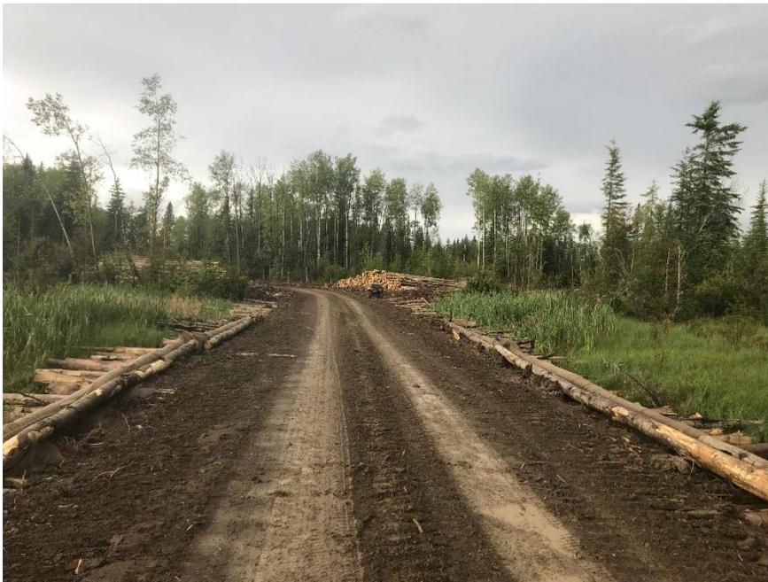
Figure 2. A typical temporary stream crossing
