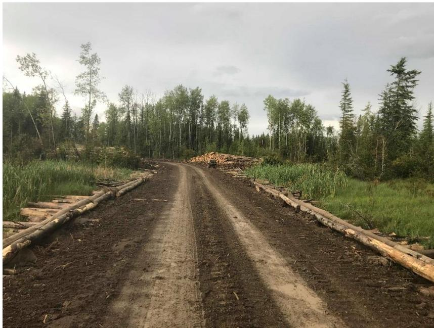
Figure 2. Temporary stream crossing in a cutblock. Modified logfill.
